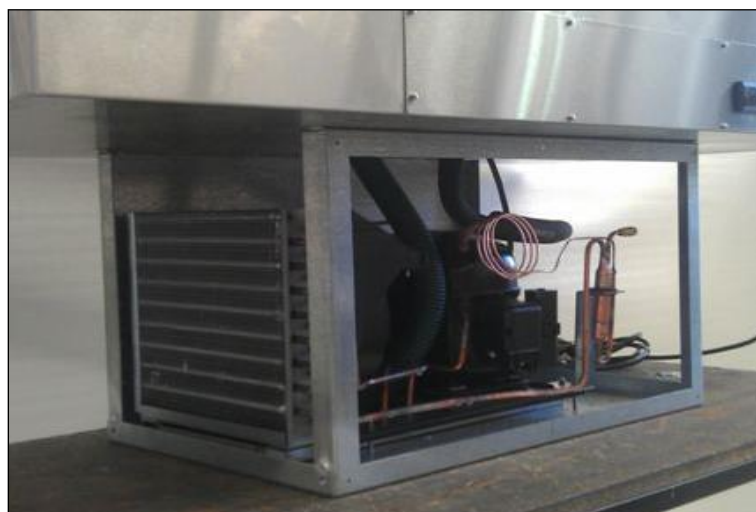
Condenser in Cradle attached under cabinet.
