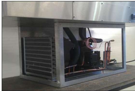
Condenser in Cradle attached under cabinet.
